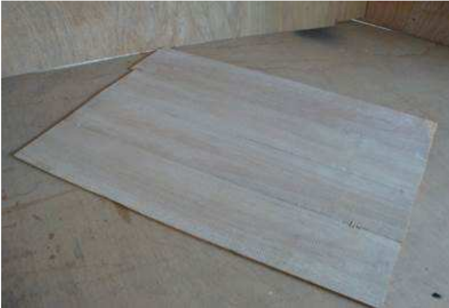
Photo 3.7.1 Boards of the soundboard are adjusted & glued altogether.
